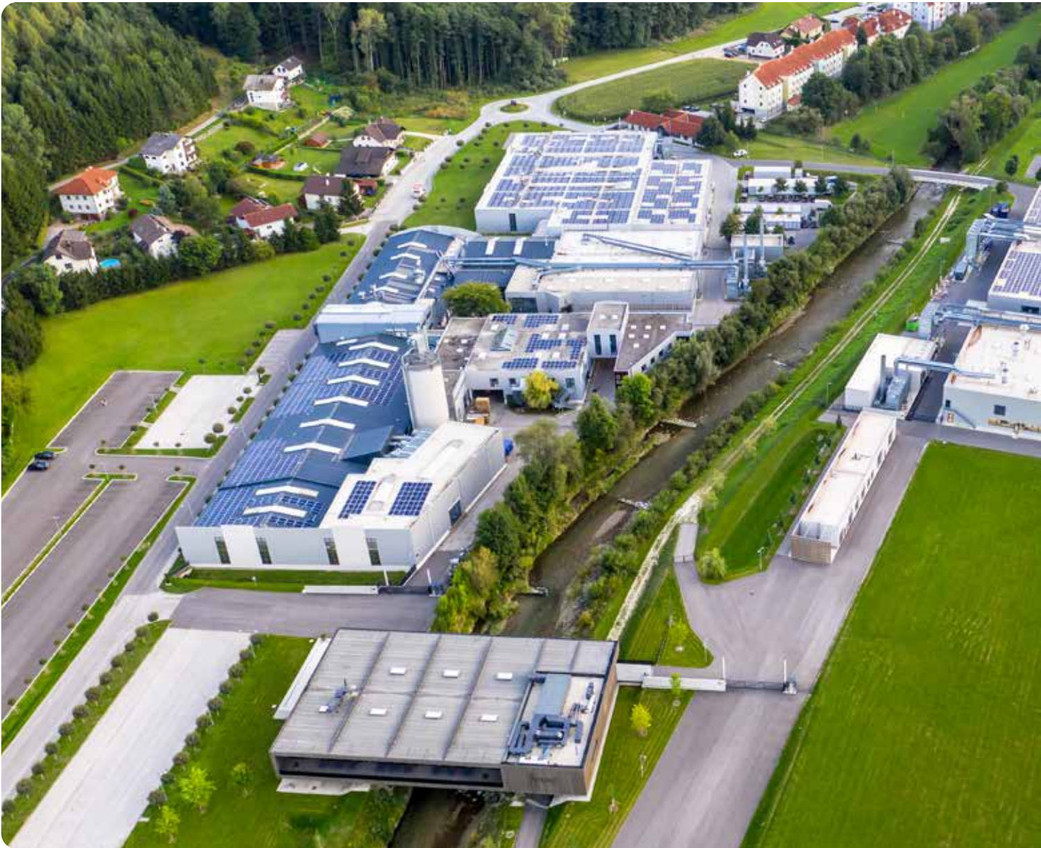
The Thomasberg facility features an extensive photovoltaic installation
