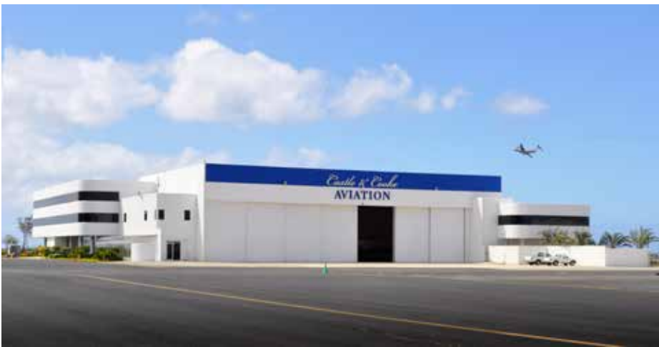
Above: Hangar and FBO facilities at Castle & Cooke Honolulu
